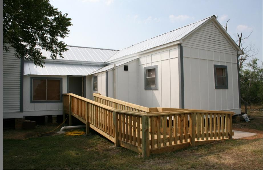
Installed new roof, ramp, window, electrical service panel, painted interior, & exterior
